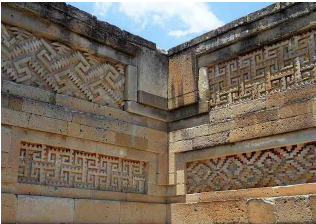
Mitla: Stone Mosaics Set in Adobe to Counter Damage from Earthquakes
